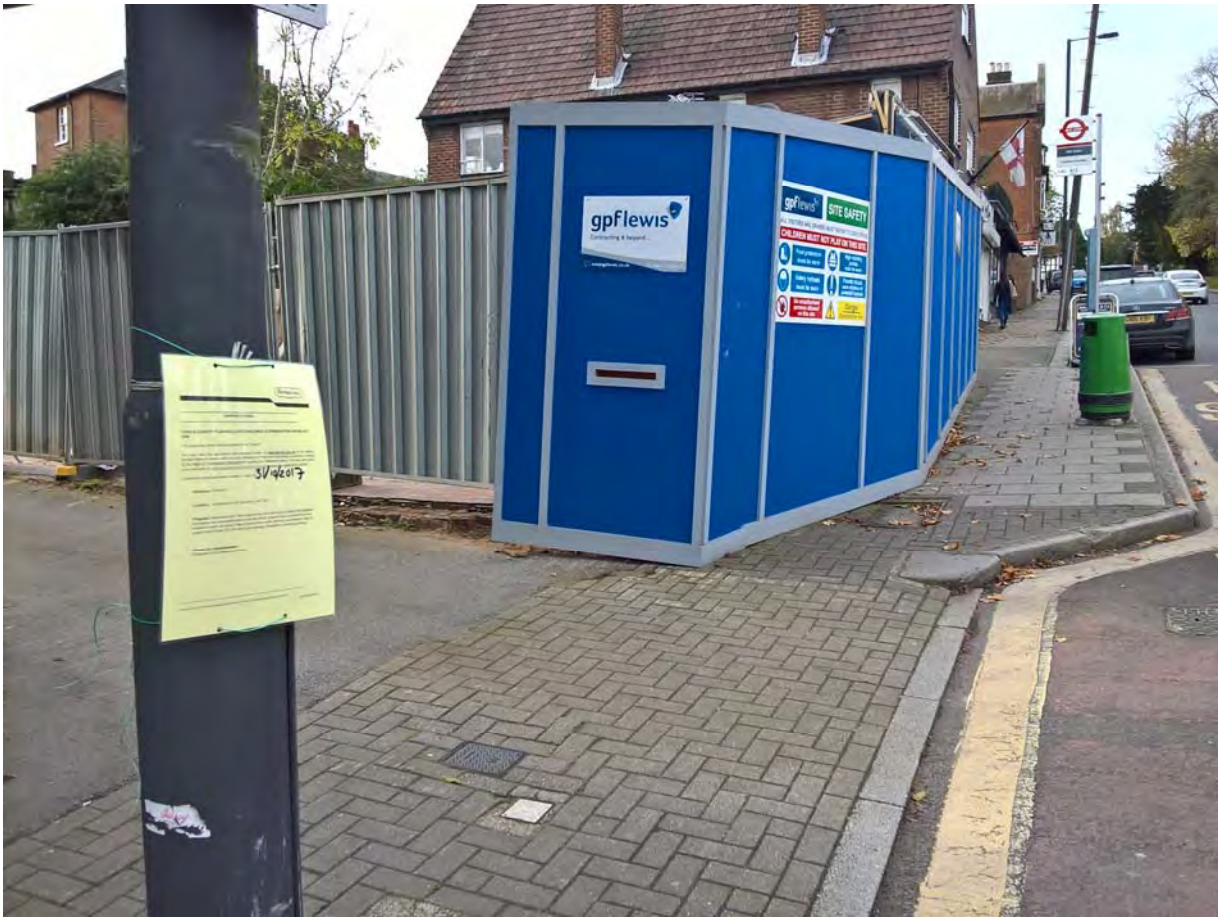
Front/side of cleared site from Stanmore Hill
